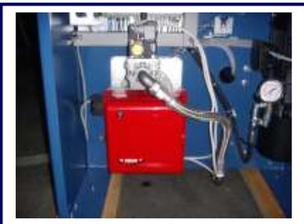
When there is a **modulating burner (BS3/M)** installed, the **lowest possible power output must be regulated below 60kW !!!** This to ensure that the CO value will not be too high. (for safety reasons).
